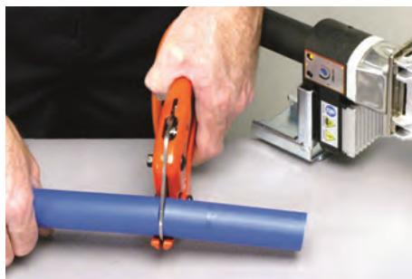
1. Turn on welder. Do not attempt welding unless tool is up to temperature (250°C). The indicator LED will cycle on/off with thermostat control when temp is correct. Cut pipe to length with approved cutters for a square swarf-free finish.
