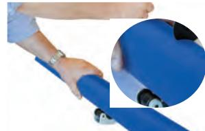
Cut pipe to length with pipe cutters for a clean swarf free finish.
